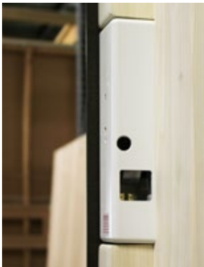
Electro-Mechanical Interlock (EMDL)
